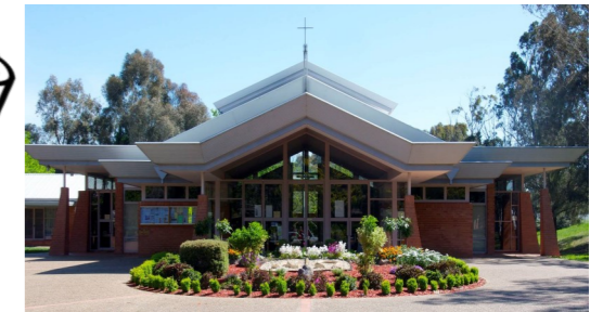
St Michael's Church Tyrrell Cct Kaleen
